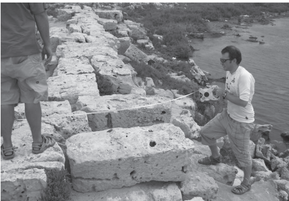
Fig. 5: The quay of Marea harbour was made of large regular limestone blocks without evidence of the use of mortar (photo: E. Khalil).
